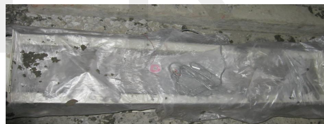
Fig.8 Beam after pouring
