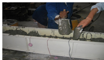
Fig.7(a) Process of concreting
