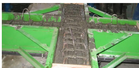
Fig. 12 Tied steel and pouring in progress
