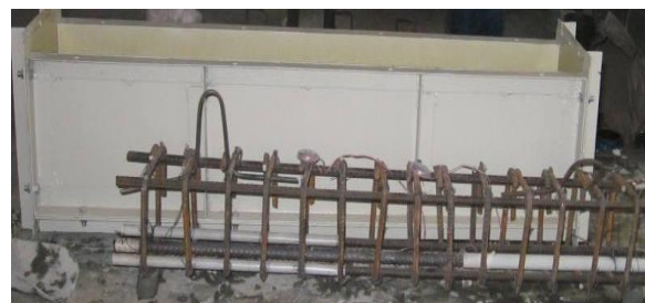
Fig.4 Tied steel with PVC pipe
