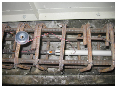
Fig.5 Tied steel with stain gauges
